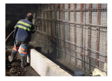
The Strata 3D Spray panels are two layers of galvanized steel-mesh on either side of an expanded polystyrene core. Designed and welded for rigid strength and flexibility, the 3D panels are easily cut to size and fastened together for a variety of construction applications. Sprayed with a concrete coating, the final structure is strong, air-tight and fire resistant. The polystyrene core maximizes flexion to absorb overpressure from blasting.
