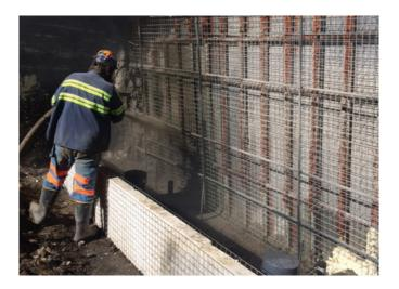
The Strata 3D Spray panels consist of a layer of galvanized steel mesh on either side of an expanded polystyrene core. The layers are welded together by diagonal inner-truss wires which create a strong and rigid structure. The 3D panels are easily joined in various configurations for mining construction and then sprayed with a concrete coating. The strength of the panels combined with the concrete layer provide an effective and air-tight structure that withstands shear force and overpressure.
